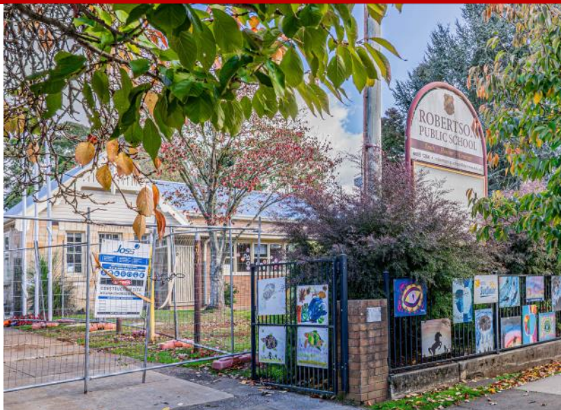
Repairs in progress—picture supplied
